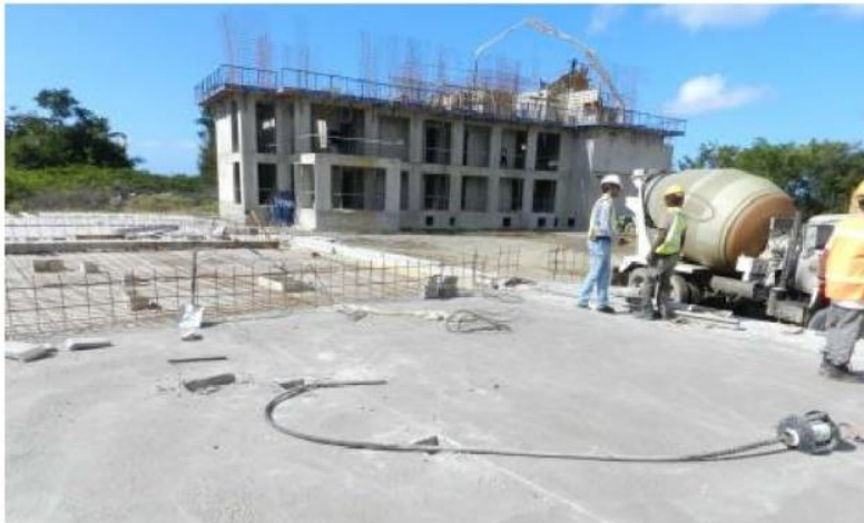
Significant progress is evident at the Cabrits Resort Kempinski in Dominica
