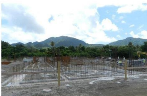
Construction well underway at the Cabrits Resort Kempinski
